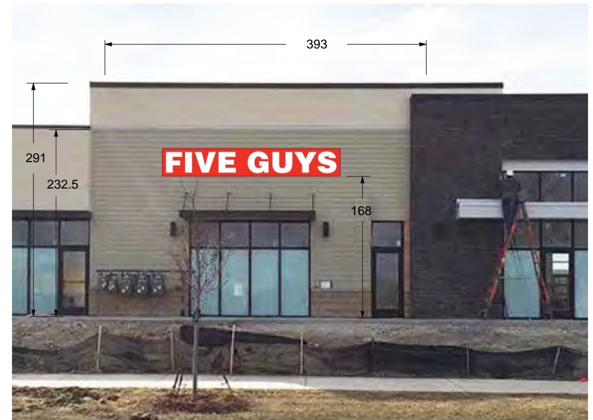
Sign in Place: South Elevation
