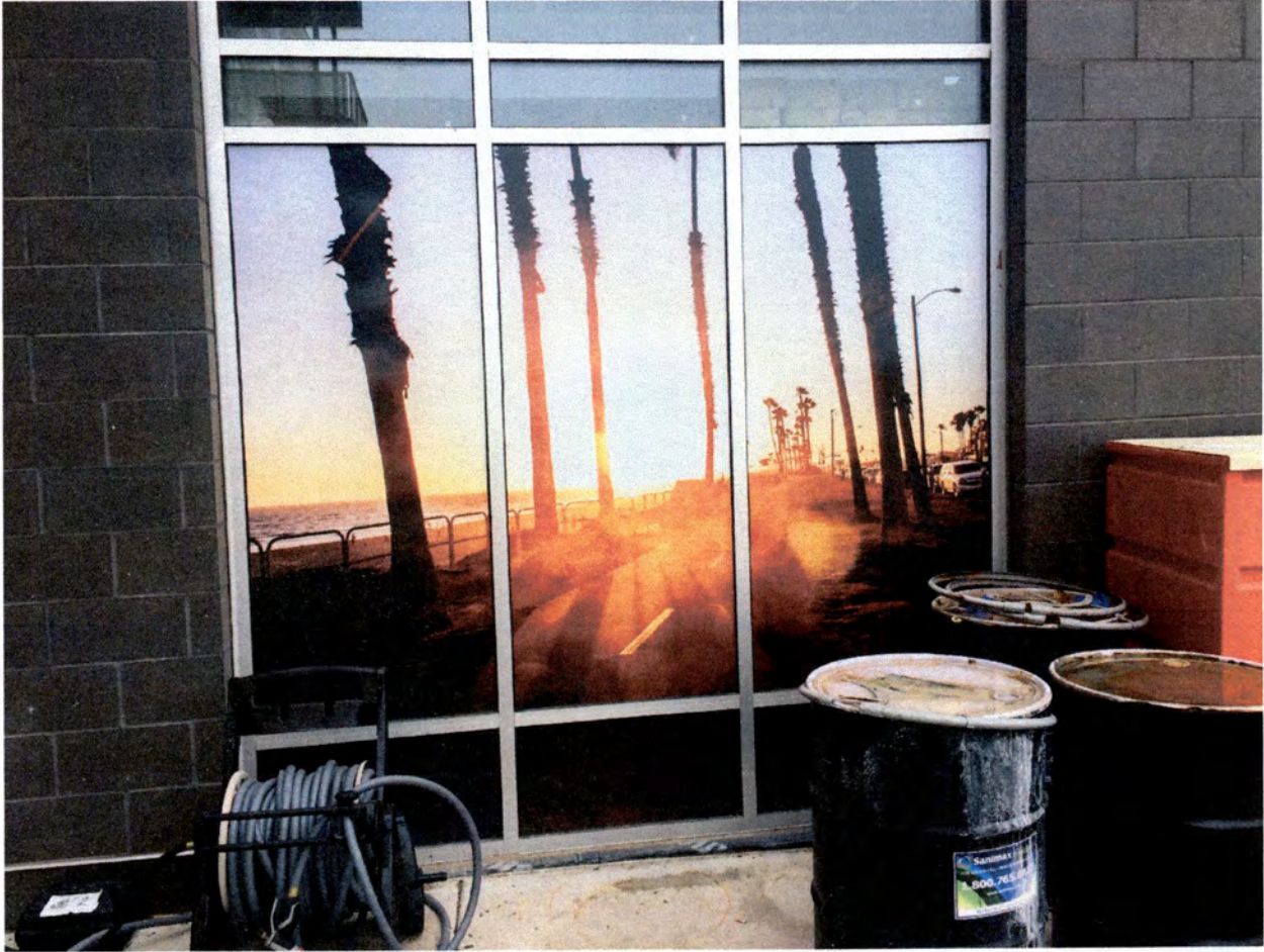
Image 6 North elevation, exterior of dry storage.
