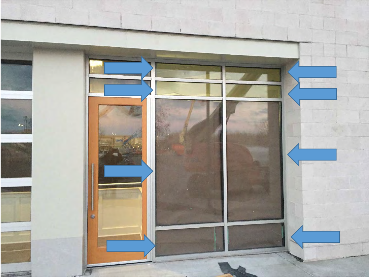
Back office area (north/northeast facing)
