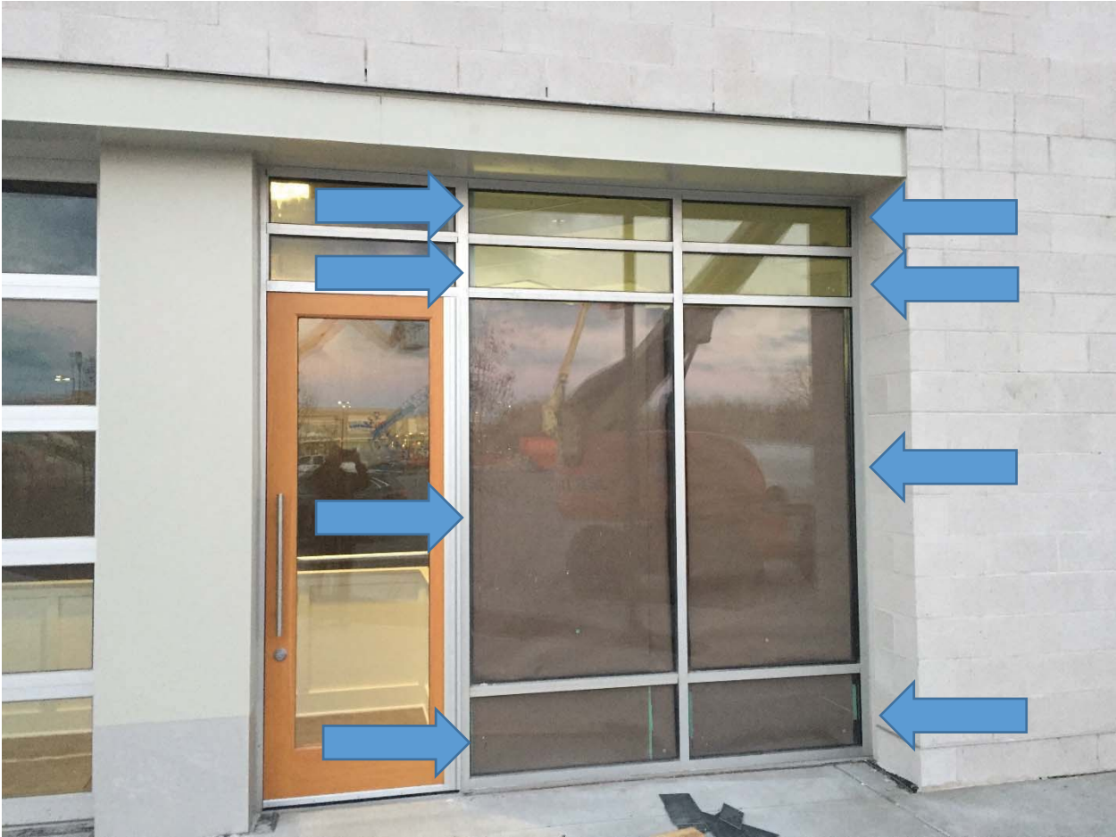
Back office area (north/northeast facing)
