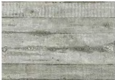
BOARD FORM CONCRETE
