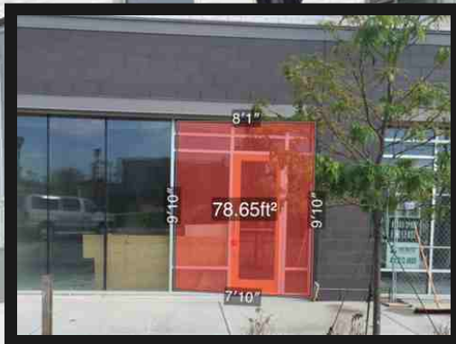
North View of Forge Building
