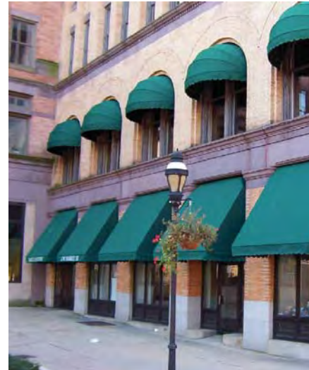
RECOMMENDED: Dome awnings complement upper arched windows. Colors are neutral and consistent. Awnings are made of durable canvas.
