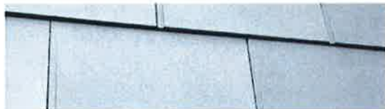
Zalmag Finish Metal Tile (for Second Floor Stair Addition) SCALE: NO SCALE
