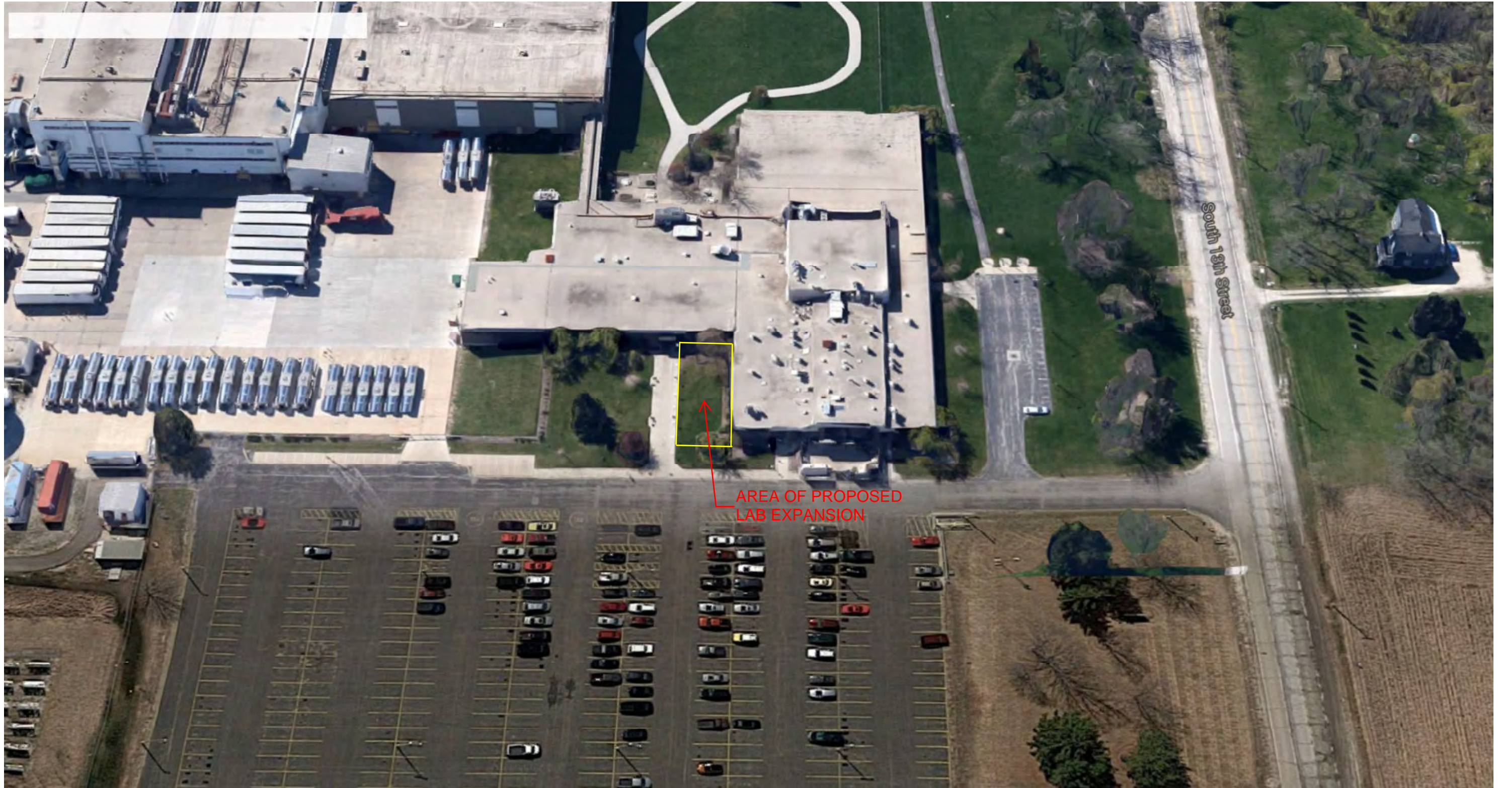
PARTIAL AERIAL PLAN LOOKING SOUTH AT PPG INDUSTRIES, INC. 10800 SOUTH 13TH STREET, OAK CREEK, WI.
