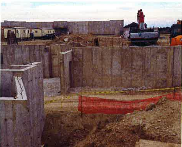
Parking garage foundation entry facing east
