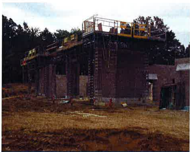
Front facing southeast
