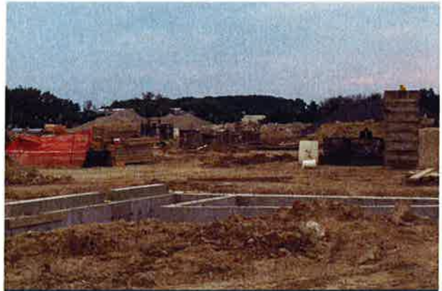
Foundation facing northwest
