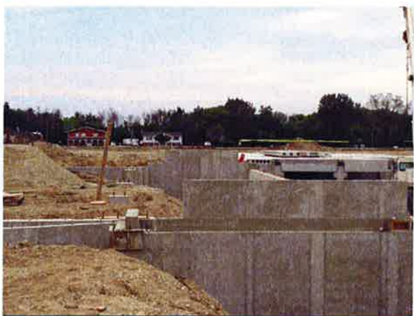
Parking garage foundation facing north
