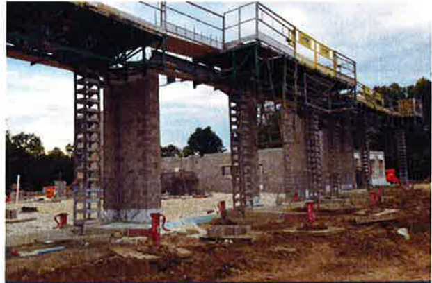
Entry to garage facing west
