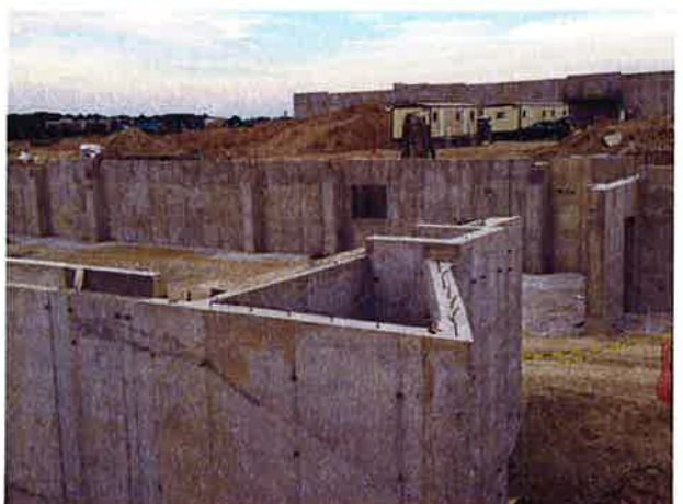
Parking garage foundation at entry
