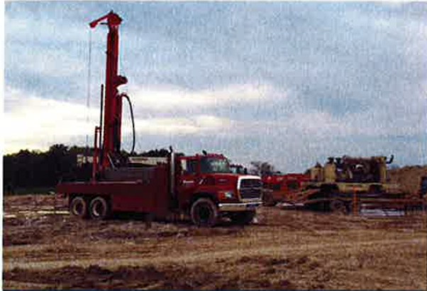
Geo thermal system drilling
