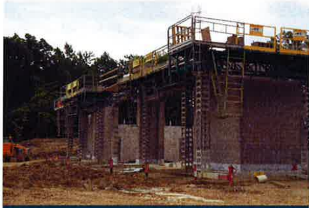
Entry to garage facing east
