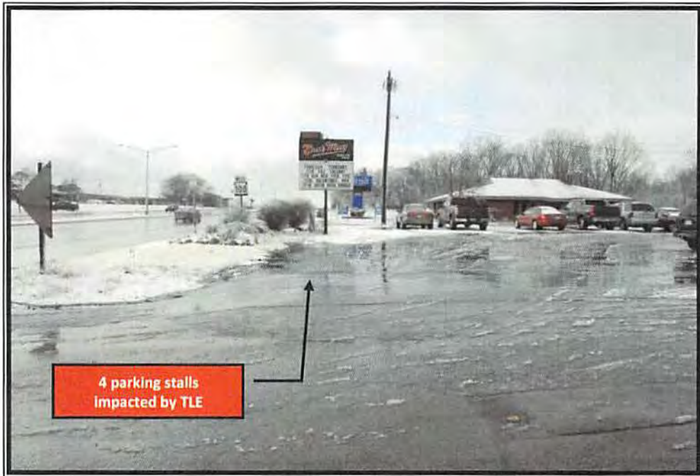
3) View of TLE and Fee Taking area looking west across property
