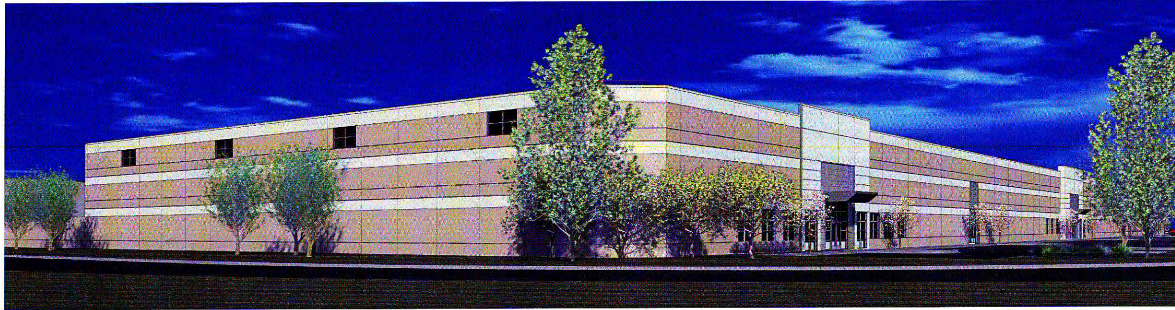
VIEW LOOKING NORTH ON REINHART DRIVE
