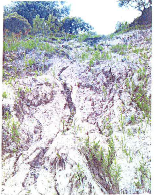
Zone 1 - Active erosion on bluff face
