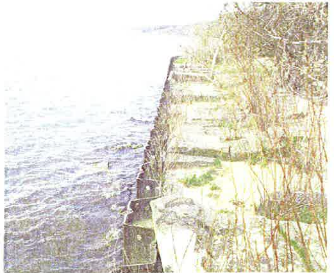
Zone 3 - Existing revetted sheet pile wall near City water intake plant
