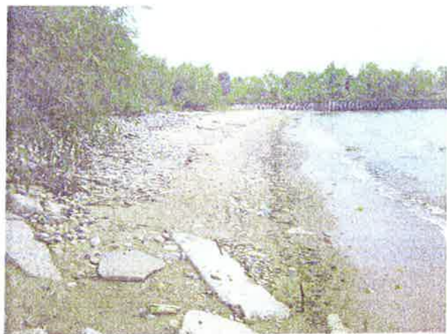
Existing beach condition along the shoreline in Zone 1
