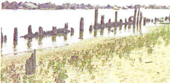
Zone 2 - Beach zone landward of existing breakwater
