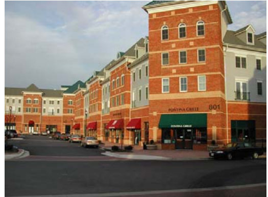
Example of a well-articulated corner building, with commercial development on the ground floor and residential on the upper floors.
