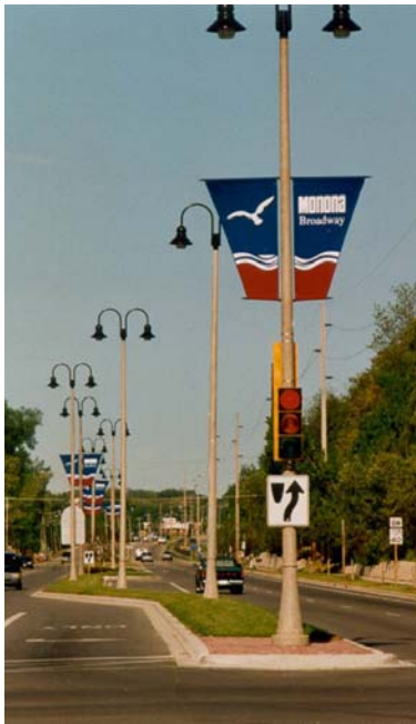
Boulevard roadway lighting and landscaping with banners and pedestrian amenities.
