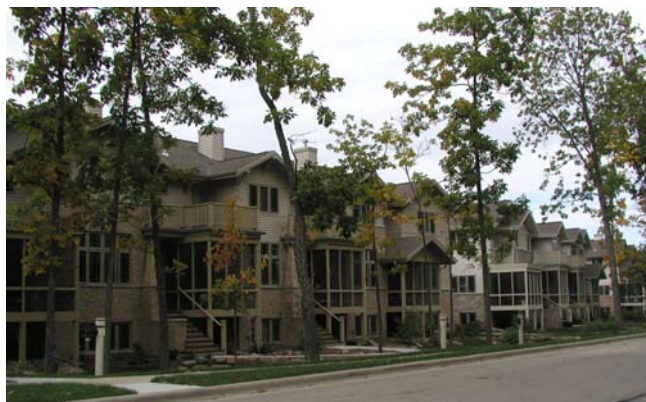
Example of a multi-family residential building with varied rooflines and façade depths, front porches and stoops.
