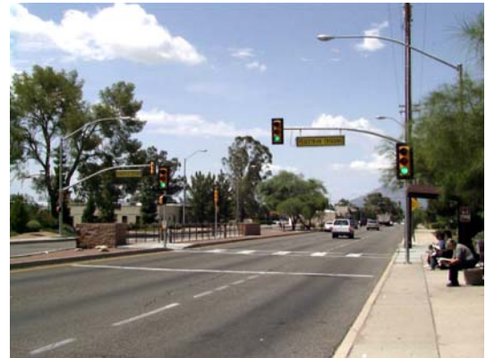
Example of a well-designed pedestrian crosswalk with refuge island, clearly defined crosswalk area, and pedestrian crossing lights.
