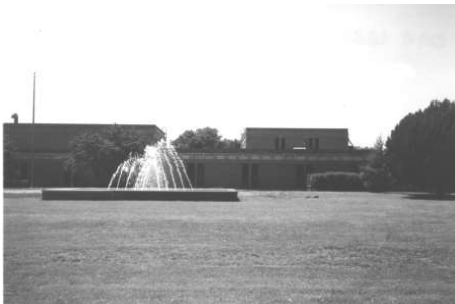
Oak Creek Water Treatment Facility
