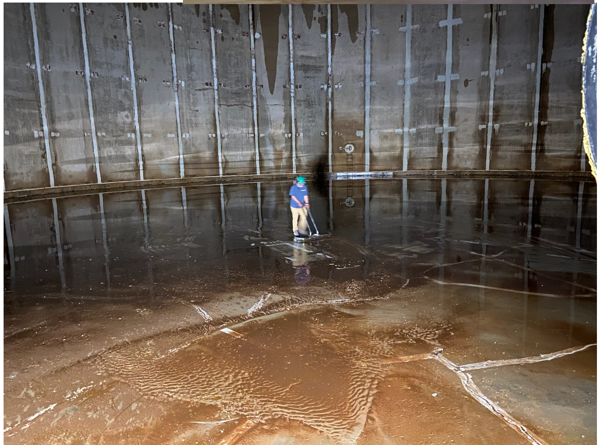
Cleaning inside the reservoir:
