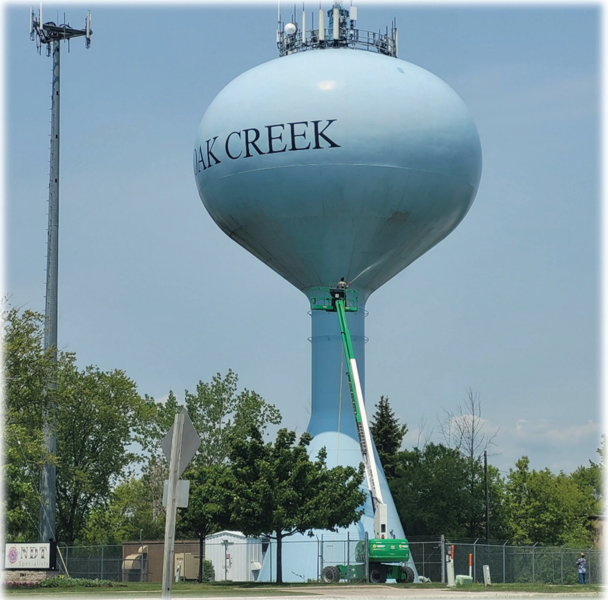
Howell Tower Cleaning
