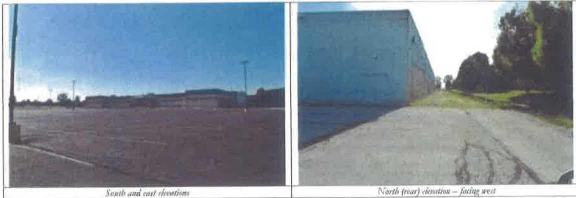
South and east elevations
