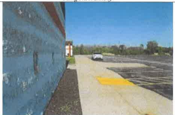
Facing east on south elevation
