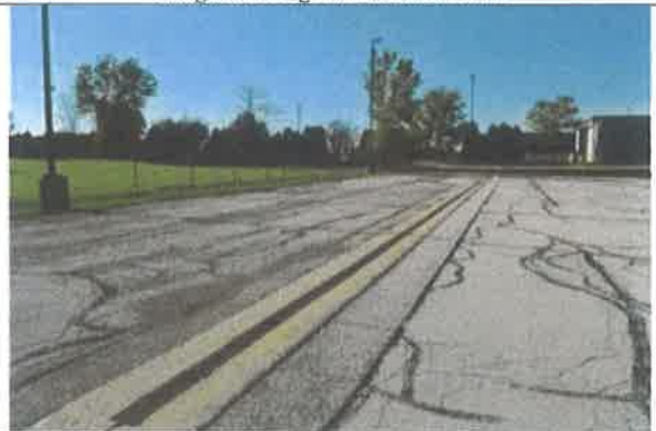
Drain in parking lot
