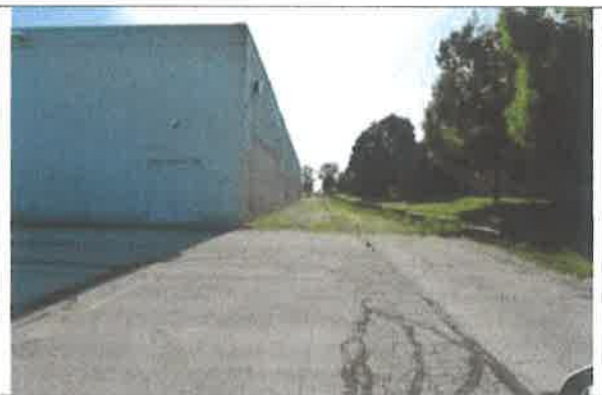
North (rear) elevation – facing west
