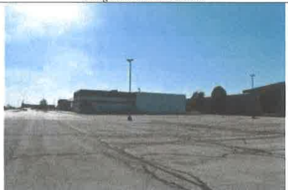
Facing west showing south and east elevations
