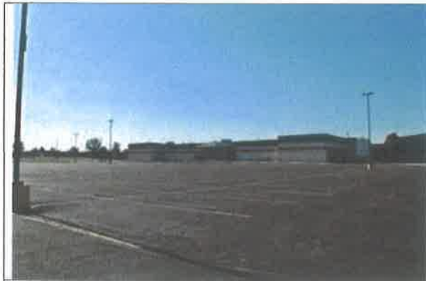
South and east elevations
