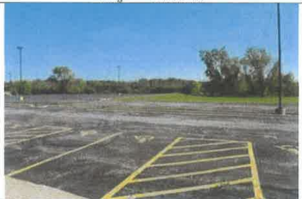
Facing southeast/south on south elevation
