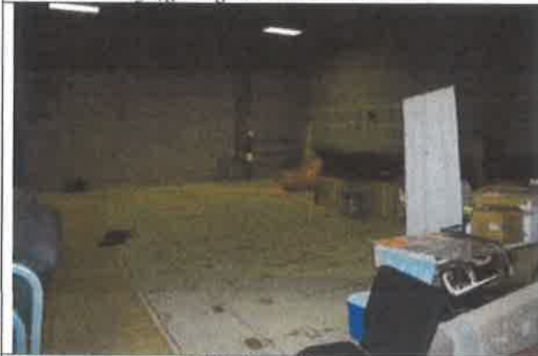
Unfinished former theater space
