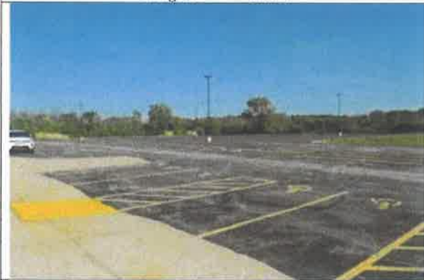
Facing southeast on south elevation
