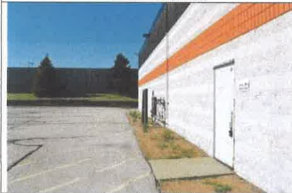
Facing north on west elevation
