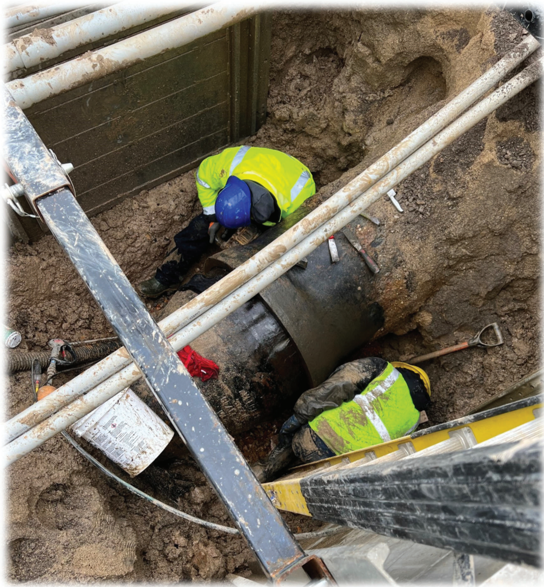
30-inch Water Main Repair
