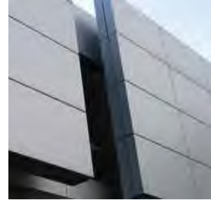
COMMERCIAL GRADE ARCHITECTURAL METAL PANEL
