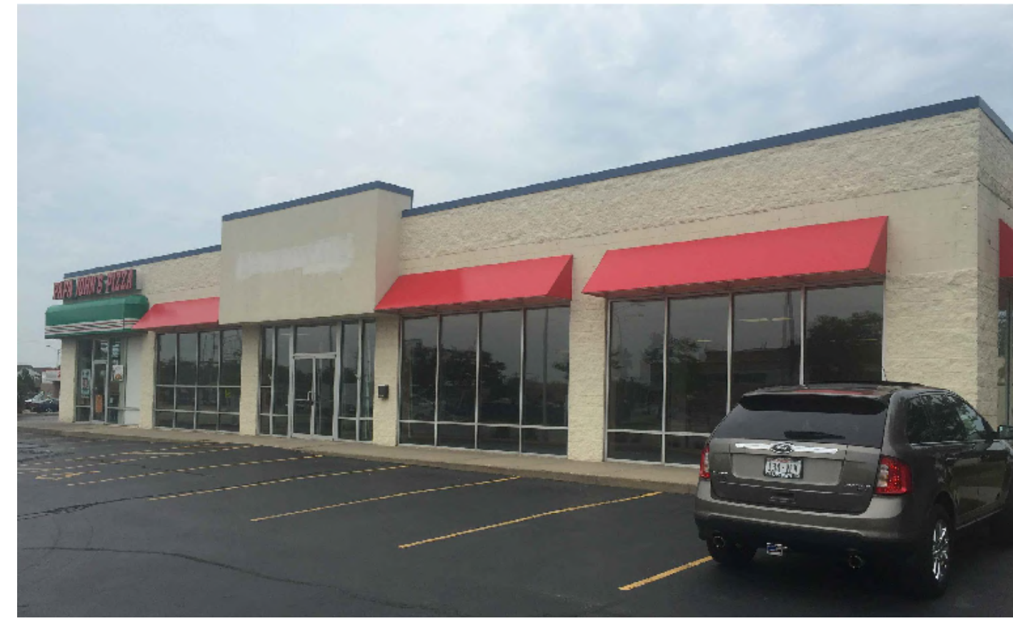
8 EXISTING EAST FACADE BUILDING PHOTOGRAPH SCALE: NONE
