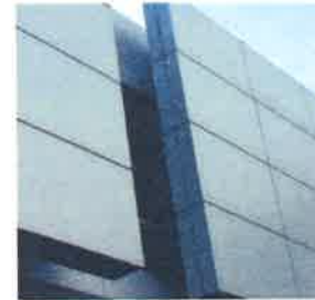
COMMERCIAL GRADE ARCHITECTURAL METAL PANEL
