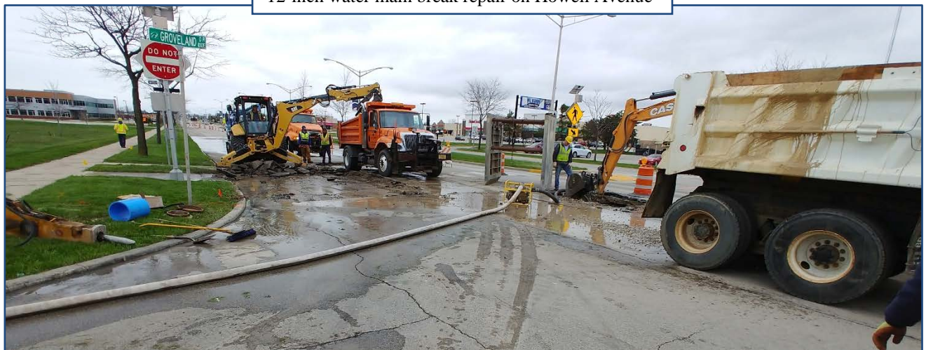
12-inch water main break repair on Howell Avenue
