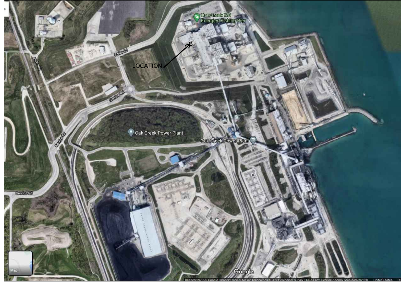
OVERVIEW- EXISTING PLANT
