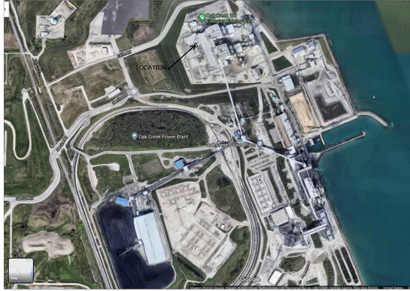
OVERVIEW- EXISTING PLANT
