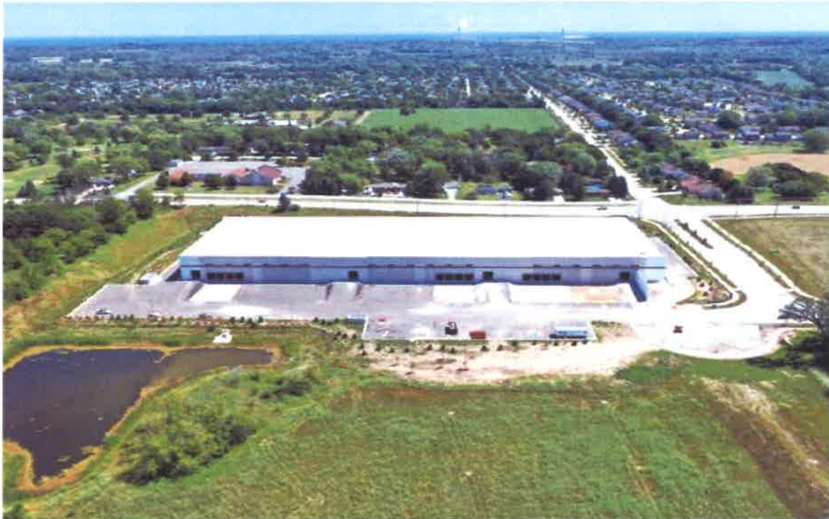
Aerial View (West looking East)
