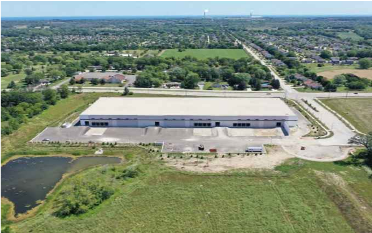
Aerial View (West looking East)
