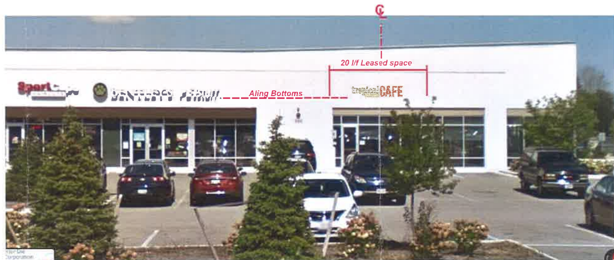
Rear Elevation @ Parking lot
