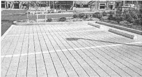
Example of permeable paving integration
