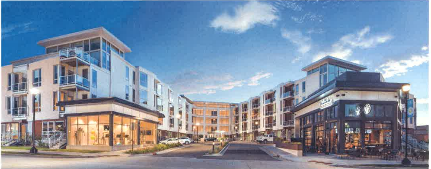
Example of successful exterior material integration
