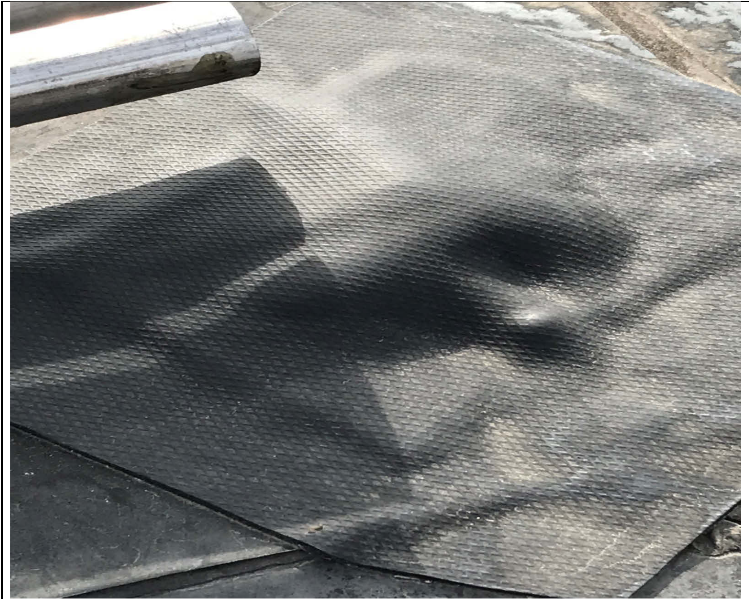
Temporary roof repair from ice damage.
