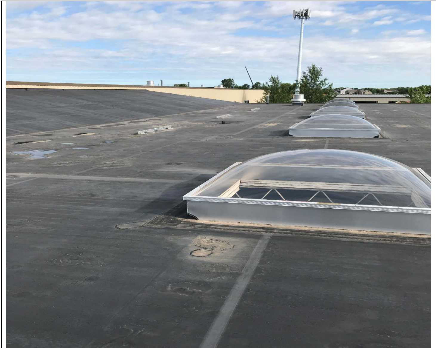
Sloped roof with existing snow rails and skylight
