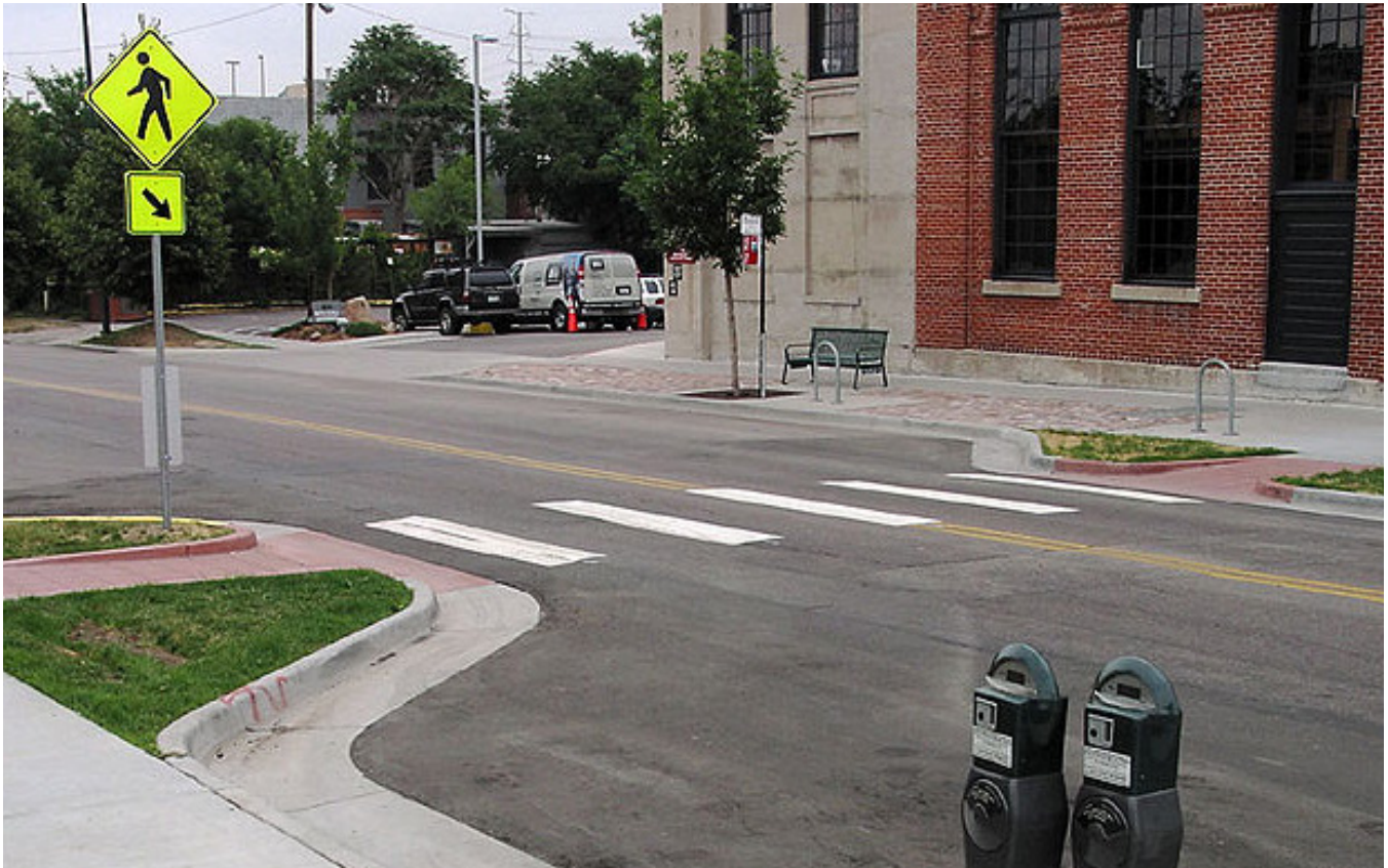
A Curb Extension / Bulb Out reduces the crossing distance. Image courtesy of emersongarfield.org
