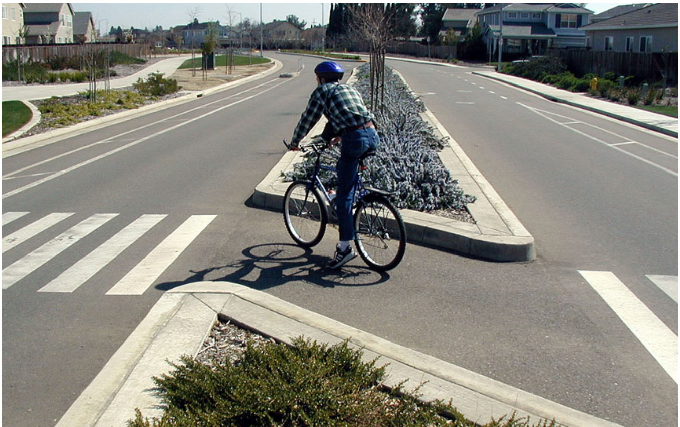
Staggering the crosswalks allows pedestrians to view the oncoming lane before continuing across. Image courtesy of Dan Burden at bikepedimages.org
