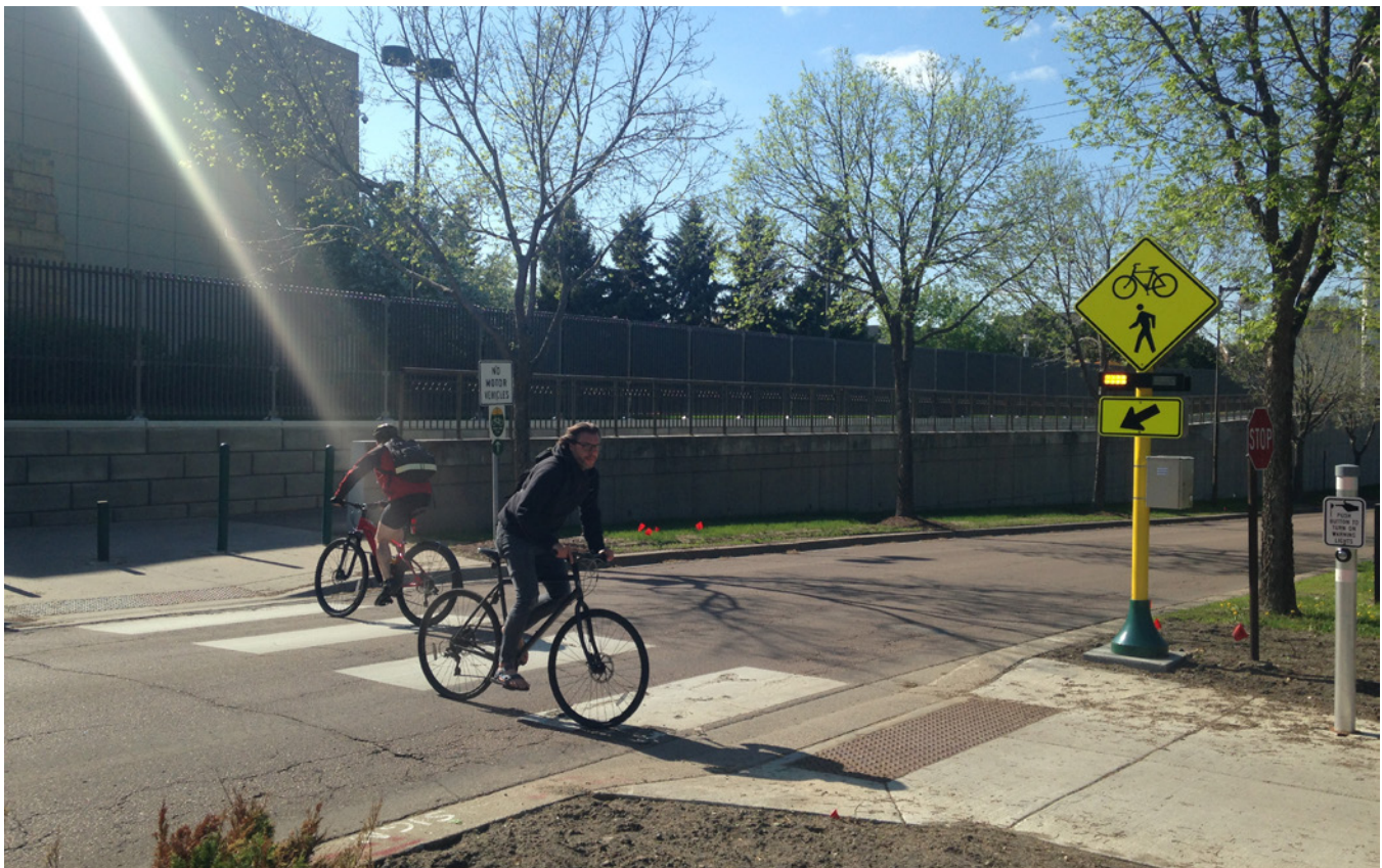
A Rectangular Rapid Flash Beacon announces the presence of bicycle riders using a roadway crossing.
