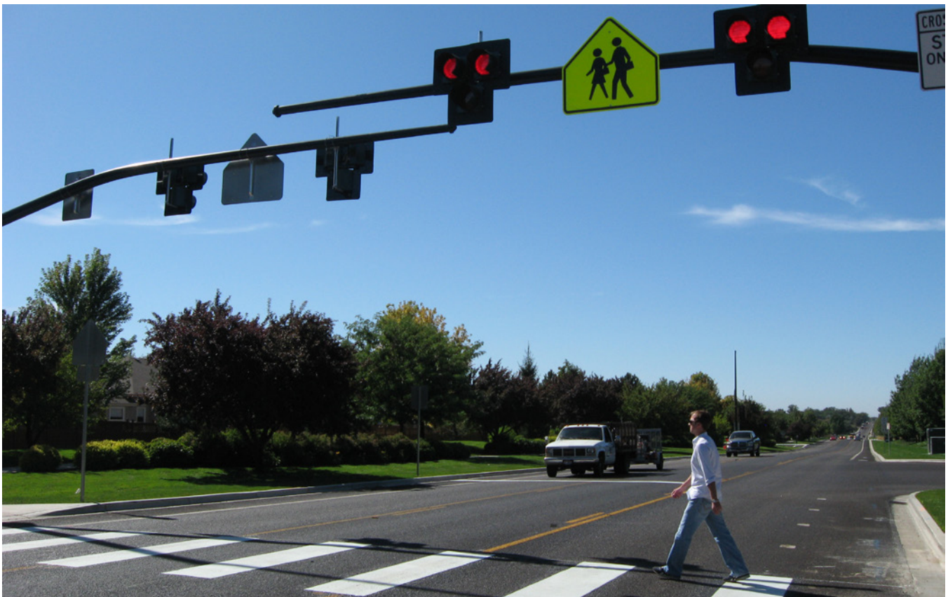
A HAWK Signal alerts motorists to the presence of pedestrians in the crosswalk.
