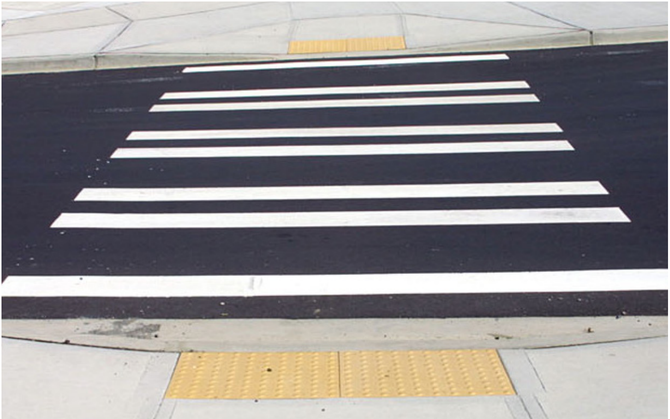
High-Visibility Crosswalks improve pedestrian visibility and crossing safety. Image courtesy of Dan Burden at bikepedimages.org
