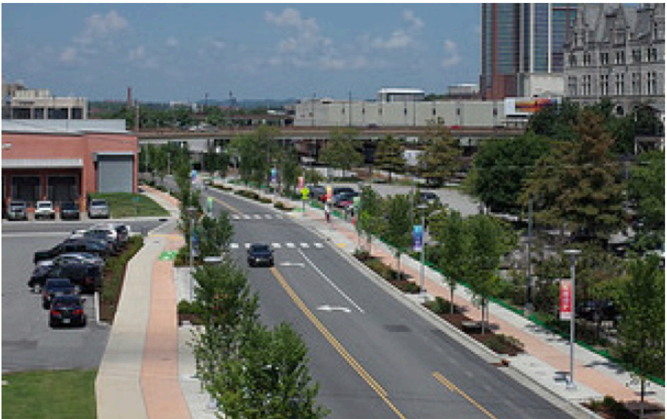
A Road Diet reallocates roadway space and improves safety for all users.
