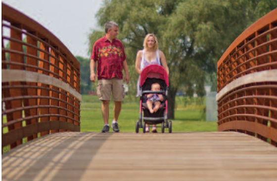
PICTURED: PEDESTRIAN BRIDGE AT ABENDSCHEIN COMMUNITY PARK
