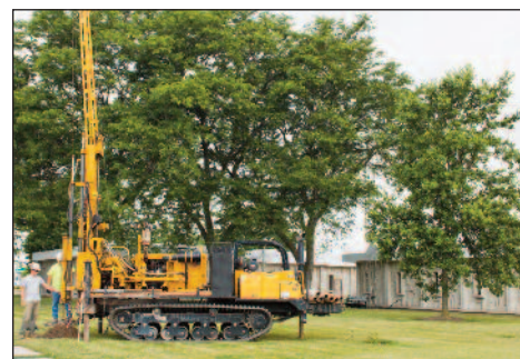
Soil boring operations at City Hall
