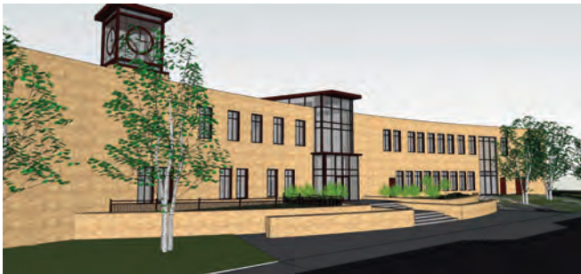
LIBRARY - WEST EXTERIOR
