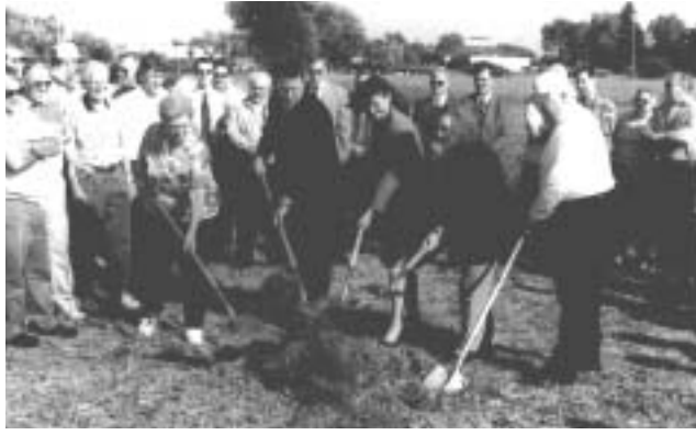
Groundbreaking for the new police station/municipal court took place on Monday, October 1, 2001. Plans to start moving ground are tentatively scheduled for early spring of 2002.
