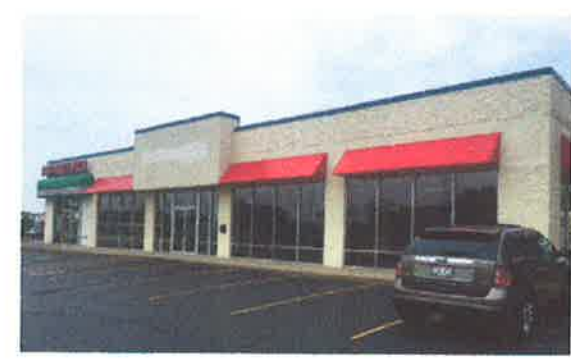
6 EXISTING EAST FACADE BUILDING PHOTOGRAPH SCALE: NONE
