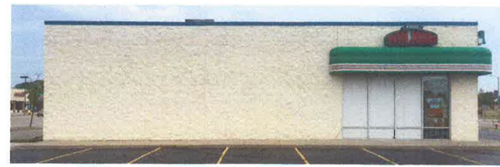
3 EXISTING SOUTH FACADE BUILDING PHOTOGRAPH SCALE: NONE
